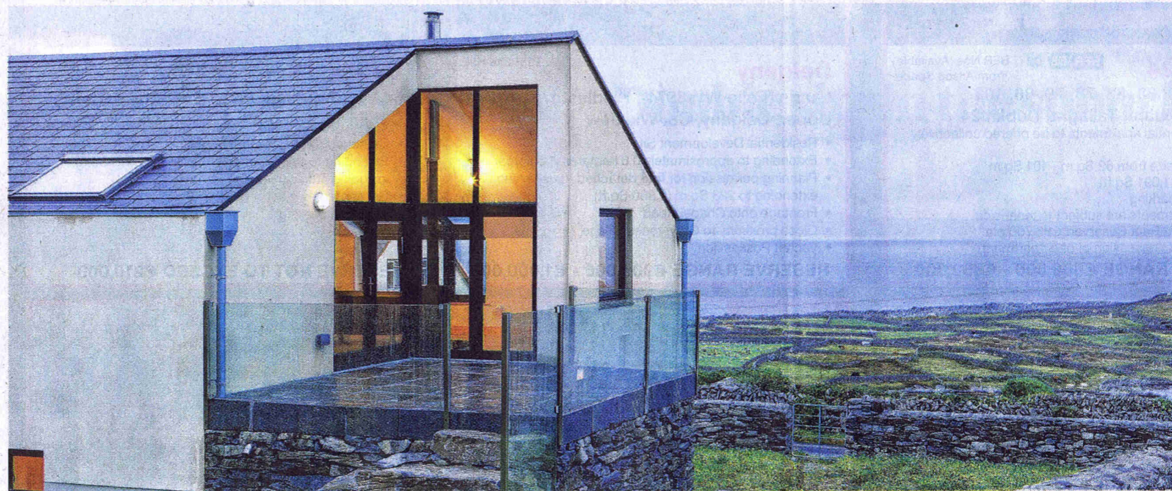
■ Brigid Keane's house on Inis Óirr, designed by architect Patti O'Neill. PHOTOGRAPH: PHILIP LAUTERBACH
